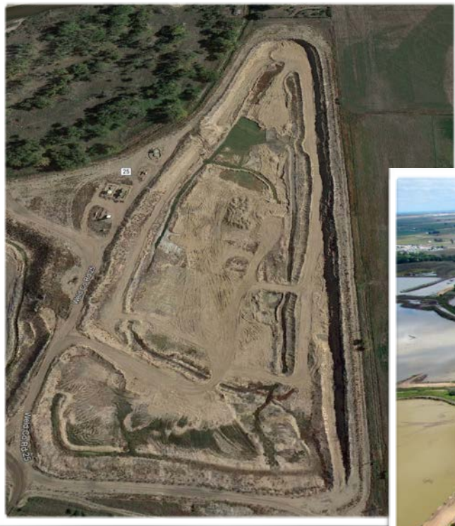
Everist Reservoir (Before)
