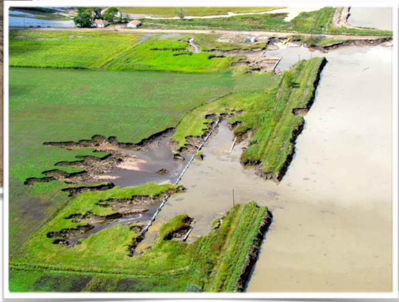
Everist Reservoir (After)
