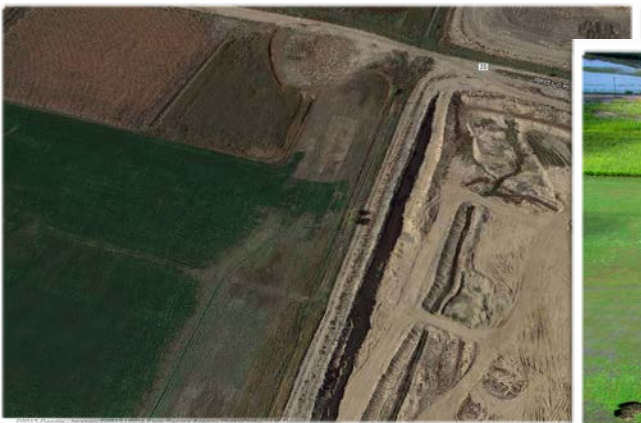
Everist Reservoir (Before)
