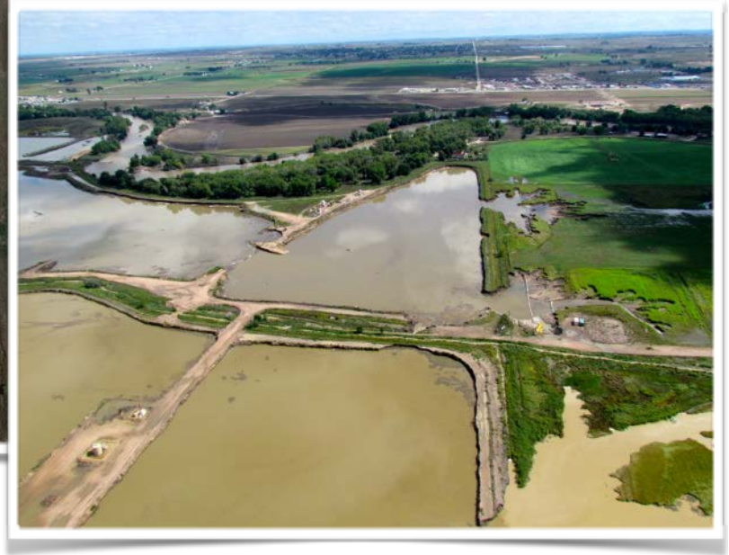
Everist Reservoir (After)
